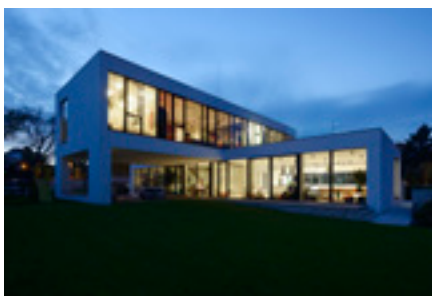
Vila ENGINE, Praha 6-Hanspaulka – SCHINDLER SEKO ARCHITECTS Jan Schindler, Ludvík Seko – 2015
