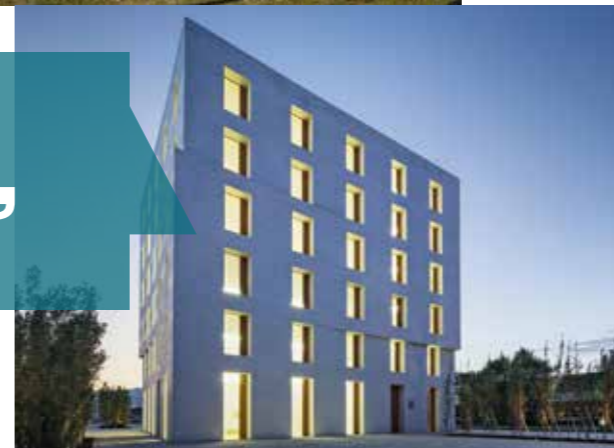
Office building (Austria) Architect: Baumschlager Eberle Photo: a rchphoto, Inc. © Baumschlager Eberle Architekten
